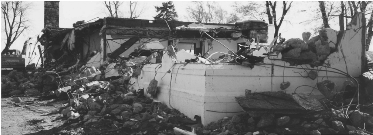
The demolition of the Old Home at October 1998.
