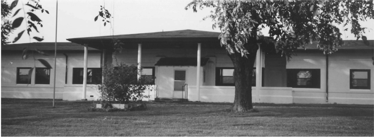
A new roof and new double-glazed windows for the Home. In 1982 Steve Miller and his friends in Northwest Indiana were actively involved with the first major renovation of the Home since 1937. The new roof provided a shady and pleasant patio for the front entrance. The new double-glazed windows were a new invention in the 1980's and they helped conserve heat in the cold winters.
