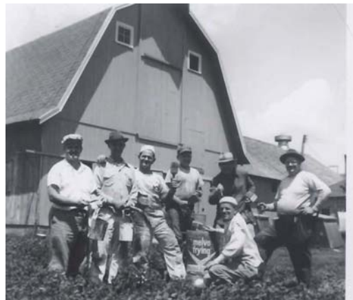
Work is finished for the happy paint crew!
